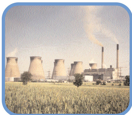
Ferrybridge Power Station, UK
