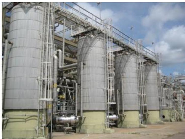
In most cases of LNG production, dehydration columns of molecular sieve desiccant are used, as this is the most effective method to reach the very low moisture content levels of less than  $0.1 \text{ ppm}_v$  moisture content required for the feed gas entering the cryogenic liquefaction process.
