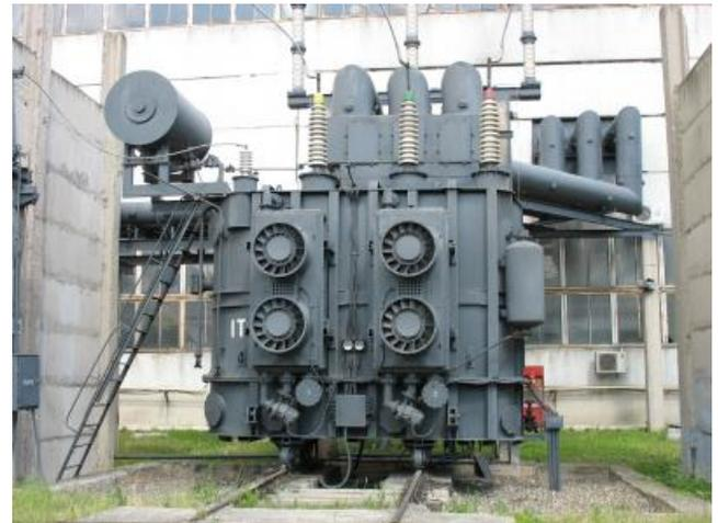
As a preventative measure, the transformer oil is replaced at regular intervals, and great lengths are taken to ensure that the water vapour content inside the transformer is as low as possible. The reasoning behind this is that moisture inside transformers adversely affects the dielectric and insulating properties of the oil.
