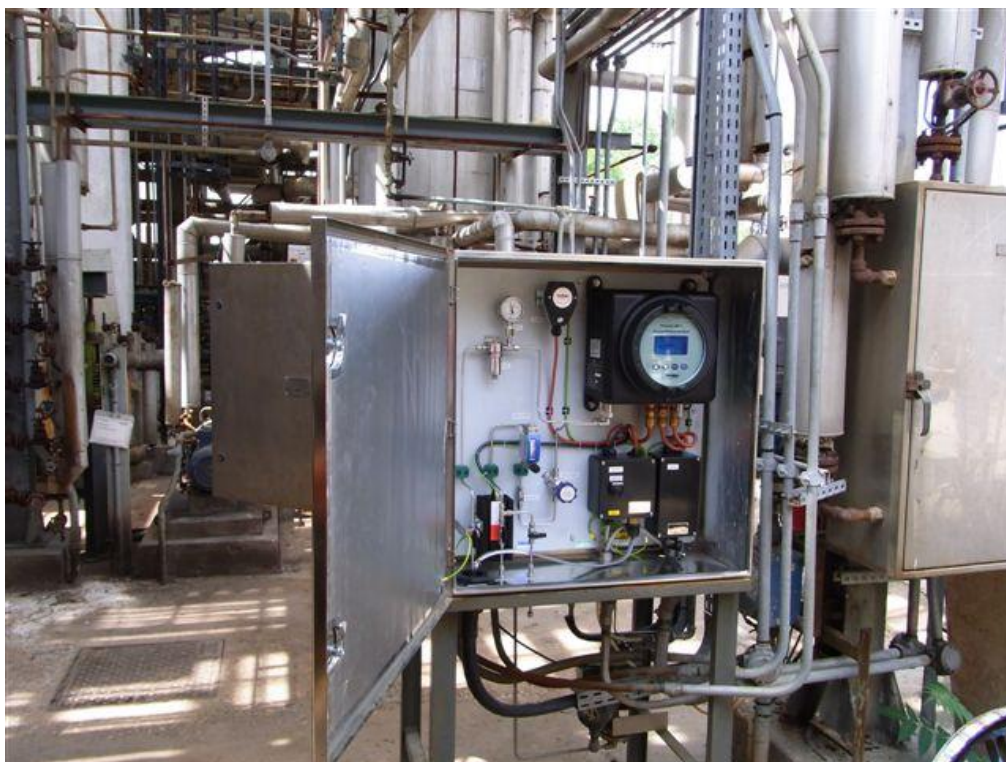
Typical installation of Promet EExd in UOP Platforming process
